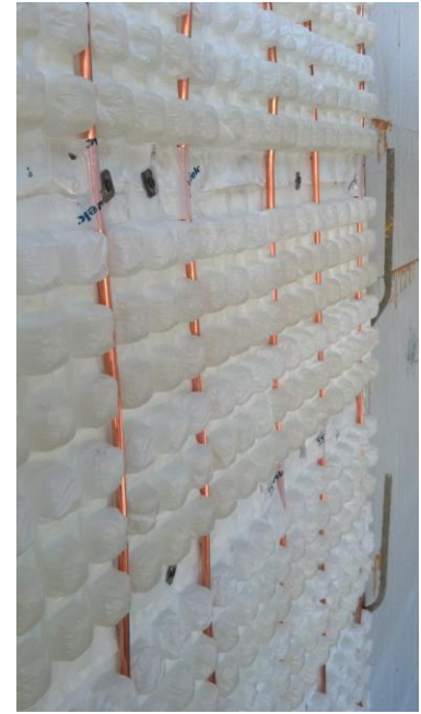
Figure 3 (a) Early DSC data for PCM and (b) the PCM mats installed with copper tubing laid over top.
