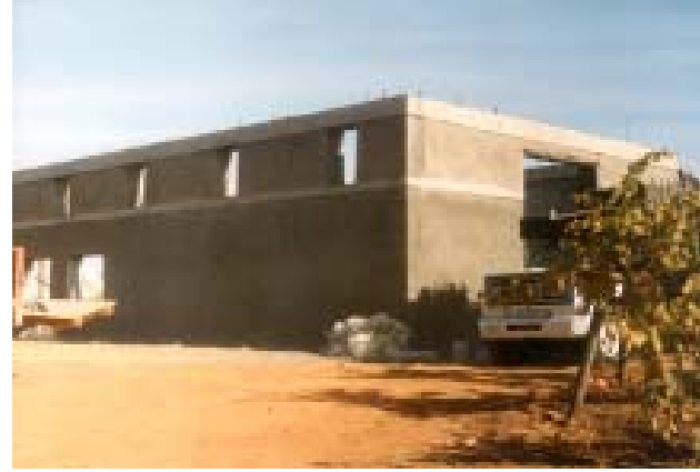
Day 10 - finished walls of winery
