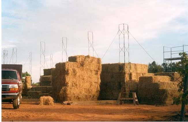
Day 1 - placing spars and bales
