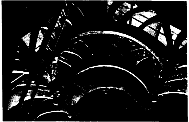
FIG. 2. Homeless Shelter, San Jose, Calif., 1989; Reinforced Concrete Roof Trusses just after Removal of Forms: Design by R. Gary Black and Chris Alexander of the C.E.S.
