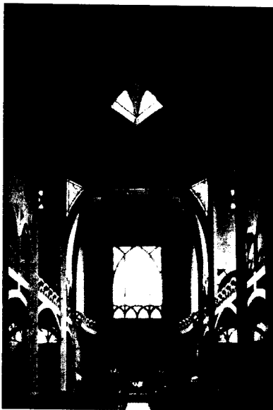
FIG. 5. Saint-Jean-de-Montmartre, Paris, 1904; Interior of Church Showing Use of Ultrathin Reinforced Cement Structure: Design by Anatole De Baudot and Paul Cottacin (Frampton and Futagawa 1983)
