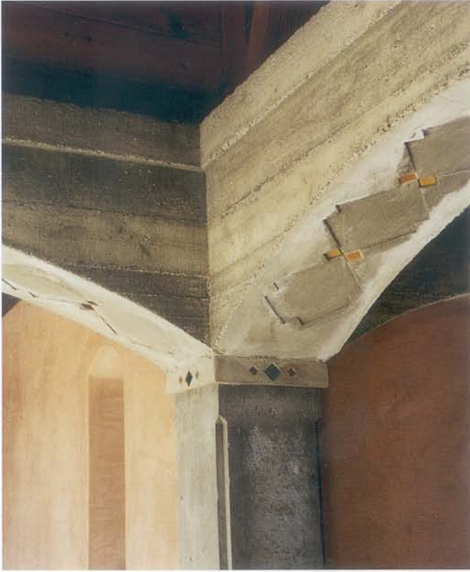
▲ Cast-in-place concrete column and arch with lacquered copper inserts give authenticity and rustic elegance to the interior.
